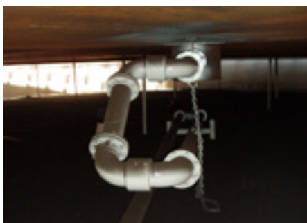
Coated carbon steel drain line arrangement.
