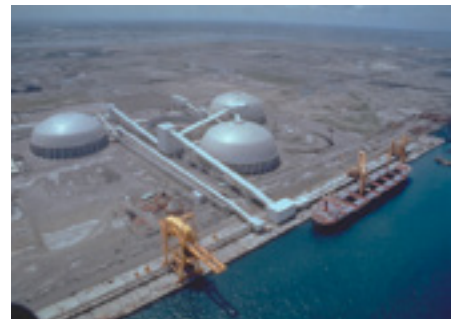
Completed 120m bulk storage domes at FPC Taiwan.
