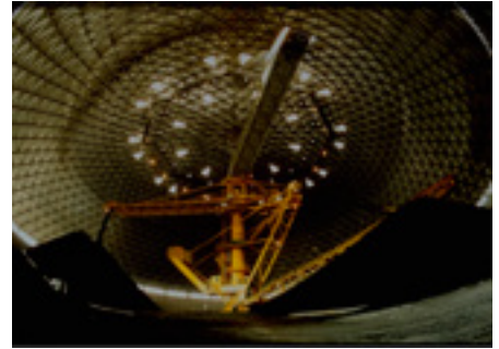
Interior view bulk storage dome for FPC Taiwan, coal storage, 120m in diameter.
