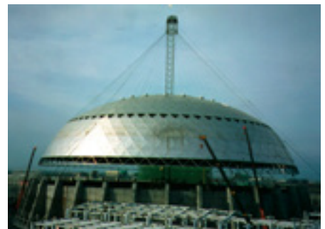
Bulk storage dome (120m) under construction at FPC in Tainwan.
